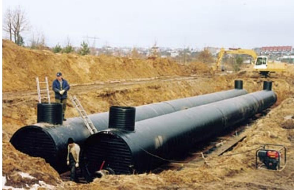
PE allow production of any manhole and fitting to order; very odd models tailor-made to optimize the properties and designs are often impossible to obtain in concrete.
