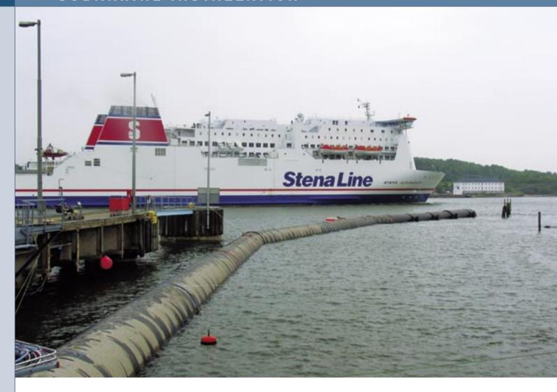
Shipping at Sweden's busiest port, Gothenburg, was able to slip in and out of the harbour without interruption when a plastic pipeline was laid just off the harbour in May. The design was exceptional in that the pipe was weighted without external concrete weights.
