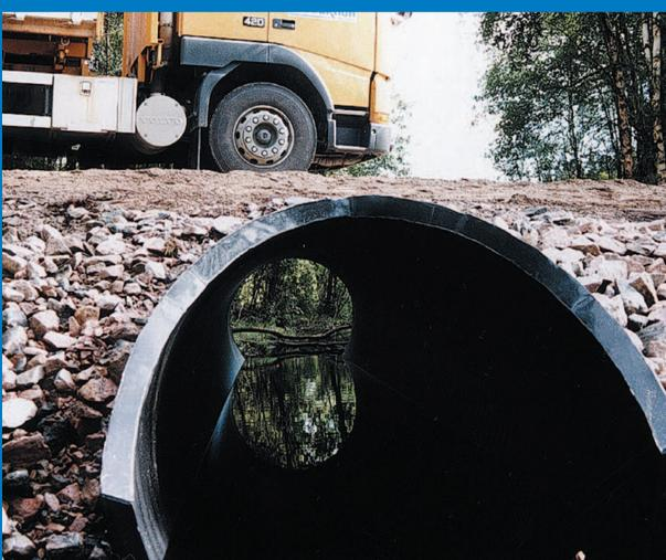
Weholite is also suitable for extending and renovating existing culverts.
