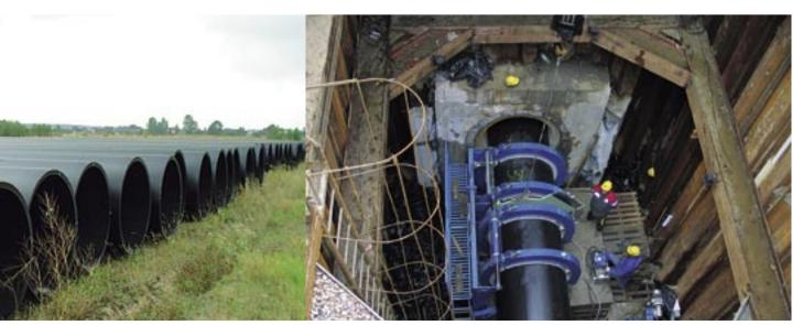
Installation of dia. 1,400 mm PE pipes in the pit under Czerniakowska St.
