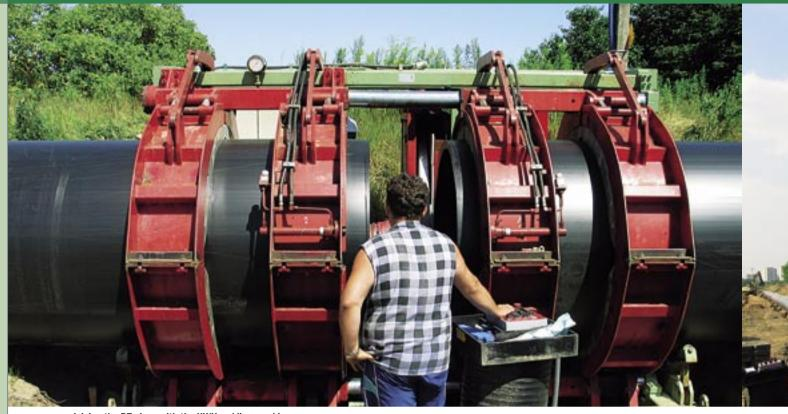
Joining the PE pipes with the KWH welding machine.
