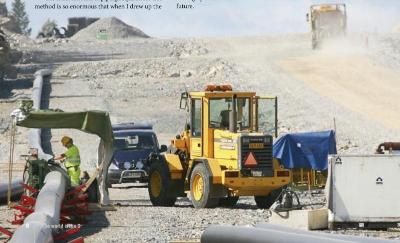
The Ämmässuo waste treatment centre, owned mainly by the Helsinki Metropolitan Area Council and the City of Espoo, Finland is currently being expanded. The new area features a service tunnel, where a collector pipeline was installed to convey runoff water from the landfill.
