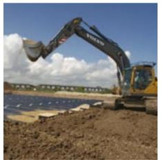
All 15 parallel Weholite pipe runs, each measuring 2,100 mm in diameter and 114 m in length, are installed. The Weholite solution is backfilled by Seymour Civil Engineering Contractors Ltd.
