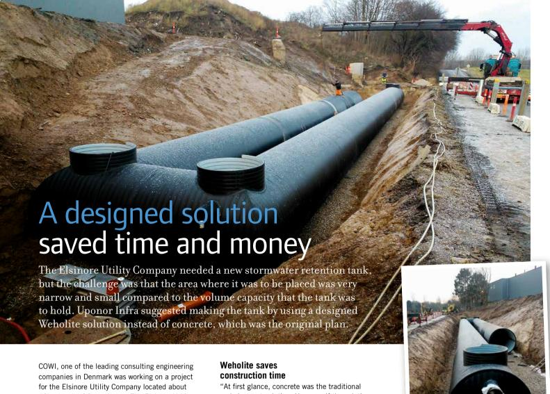
40km north of Copenhagen. The Elsinore Utility Company needed a new stormwater retention tank with a volume of about 500m3 with a maximum 31/s discharge to a nearby stream. The solution, as planned, was to use concrete, but this created challenges as this solution took up too much space. Therefore, COWI contacted Uponor to explore the possibility of using a design solution that constructed the tank out of plastic instead of concrete.
