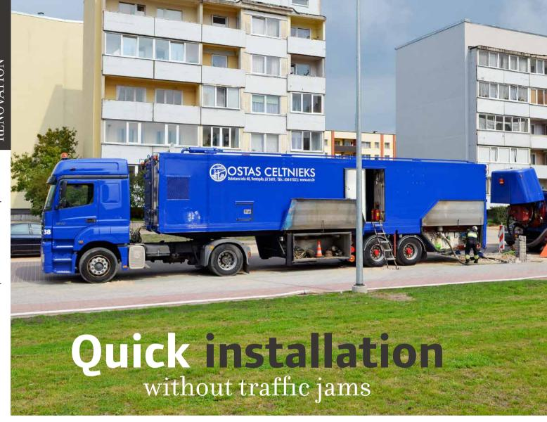
This summer for the first time in Latvia, renovation using Uponor's Omega-Liner non-entrenchment technology was carried out in two local municipalities, Madona and Ventspils, which was highly appreciated by its customers. During the 2.5km pipeline renovation the road surface was not damaged and routine traffic was affected. Renovation work was carried out quickly, avoiding the necessity to suspend service provision to clients.
